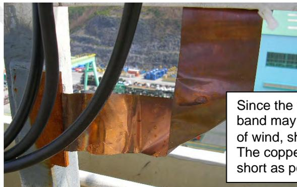
Since the welded parts of copper band may be broken by swinging of wind, shorten the copper band. The copper band should be as short as possible.
